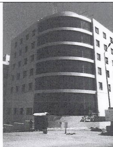
Updated View of Front Entrance to Facility
